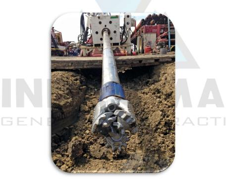
INFRAMAX General Contracting are dealing with "HORIZONTAL DIRECTIONAL DRILLING" by latest and modern technologies, capable to work on hard rocks, sand areas and under water. HDD is a steerable trenchless method of installing underground pipe, conduit, or cable in a shallow arc along a prescribed bore pass by using a drilling rig, with a minimal impact on surrounding area.
